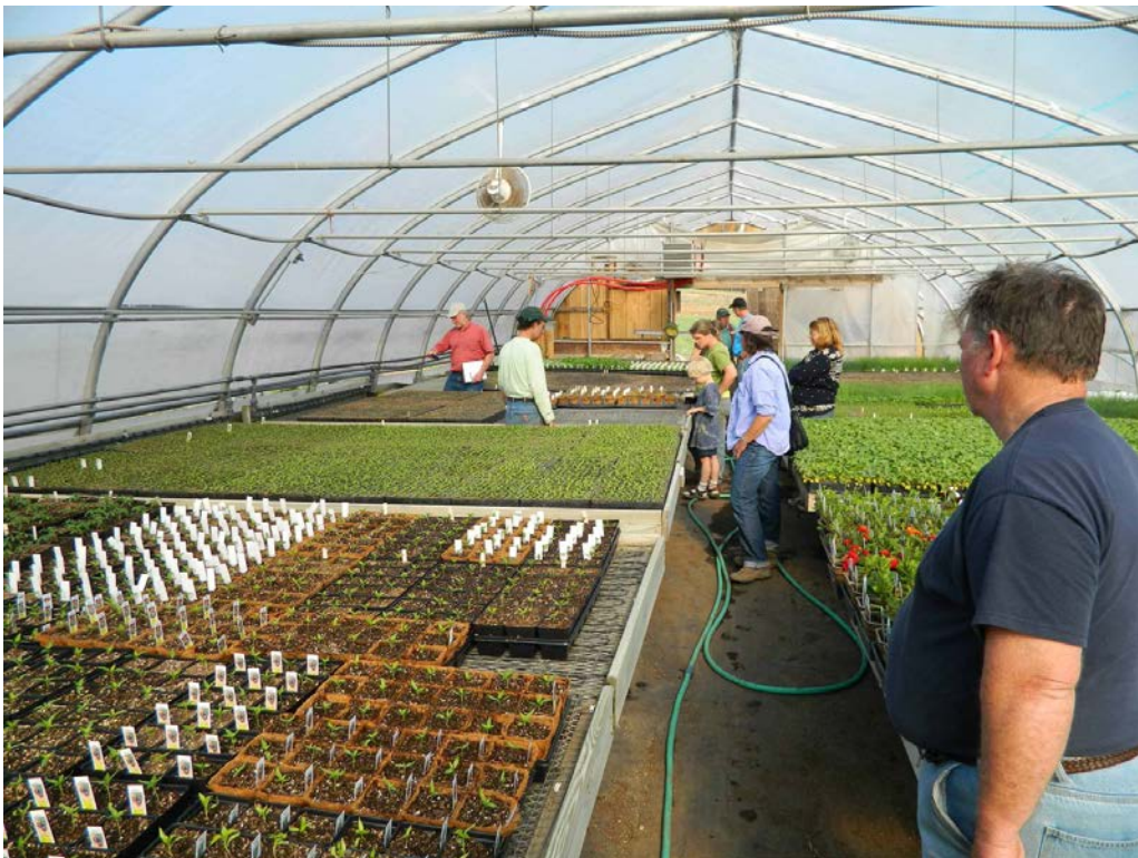
Figure 21 - Dave Marchant (Fairfax) at a later twilight meeting showing bench heating mat heated with hot water from the Maxim 250 outdoor boiler. A hydronic air heater, also fueled by the Maxim, is visible on the far end of the greenhouse.
