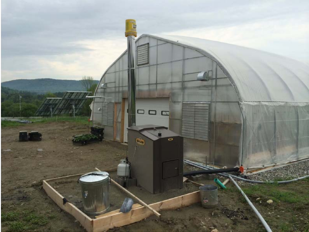
Figure 16 - A nearly completed Maxim 250 outdoor biomass boiler at Jericho Settlers Farm (Jericho).
