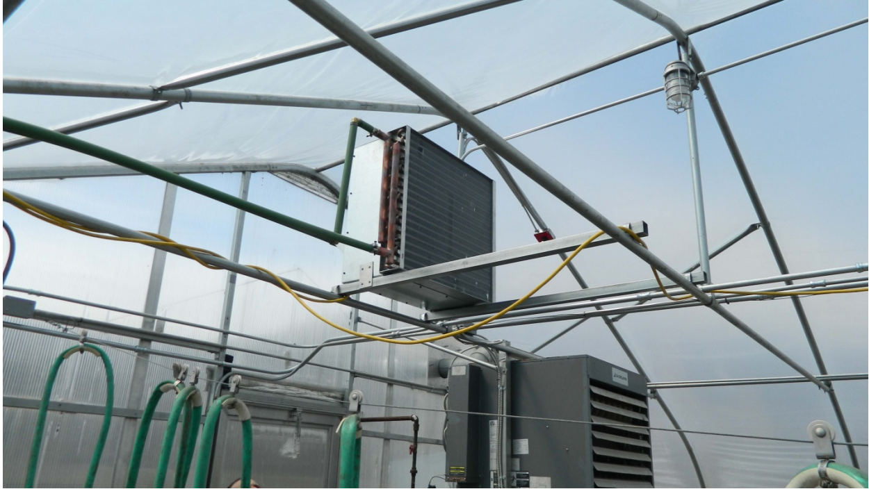
Figure 5 - Hydronic air heater at Burnt Rock Farm (Huntington).
