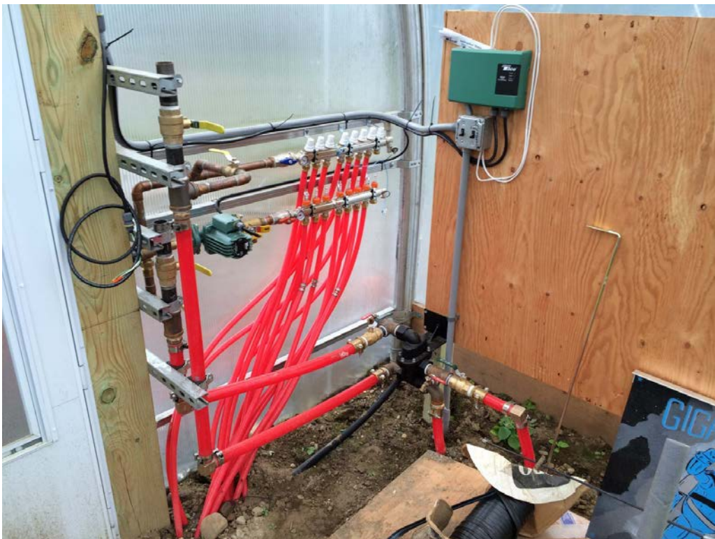
Figure 9 - Hot water manifold at Clear Brook Farm (Shaftsbury).
