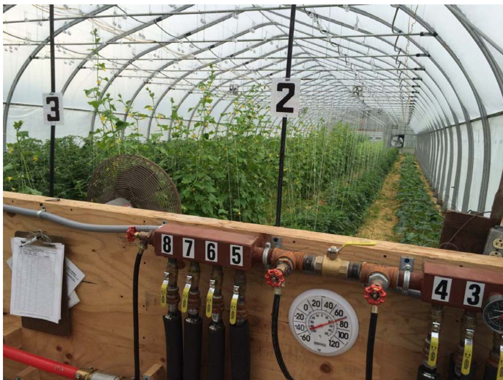
Figure 15 - Hot water distribution manifold with early cucumbers in the background at Jericho Settlers Farm (Jericho).
