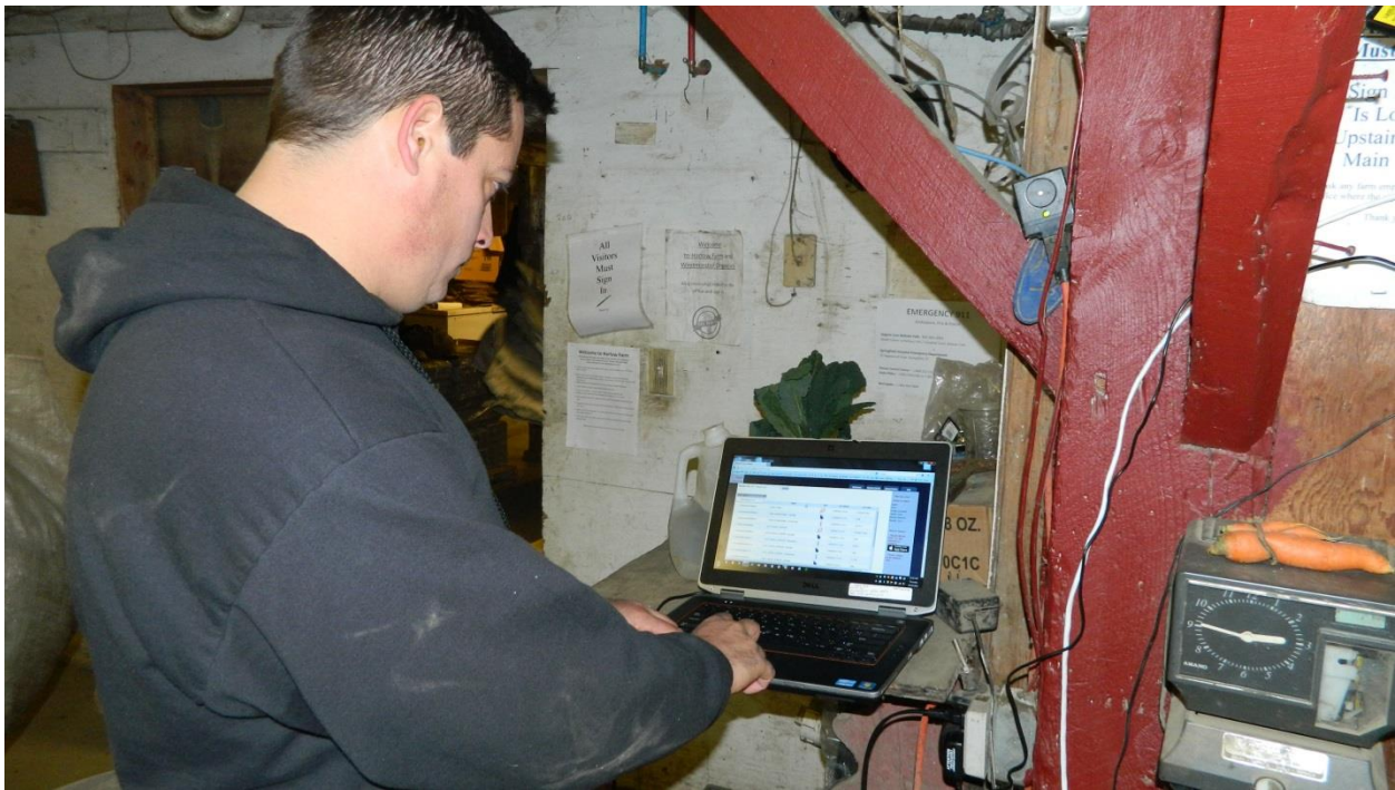
Figure 7 - Chris Callahan sets up the monitoring network at Harlow Farm in Westminster, VT. Top: Wiring the sensor network. Bottom: Checking the sensor operation via the internet.
