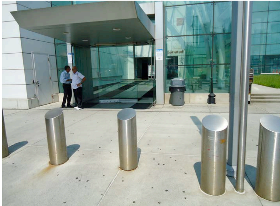
Photograph #11: Entrance Doors to Ferry Terminal
