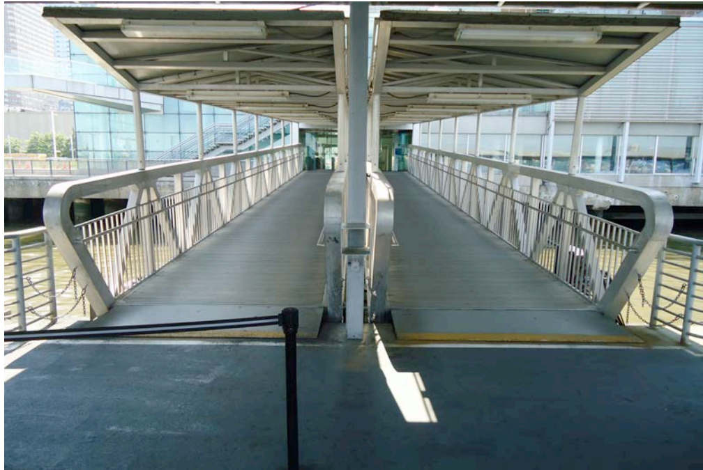
Photograph #5: Runway Connecting Ferry Terminal and Dock
