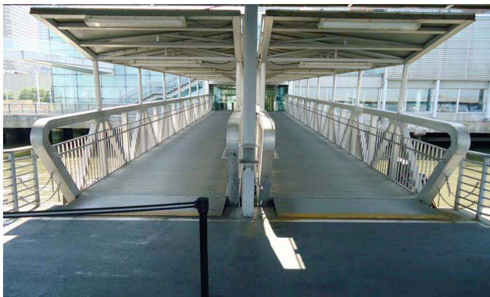
Photograph #13: Covered Ramps Connecting Ferry Terminal and Dock
