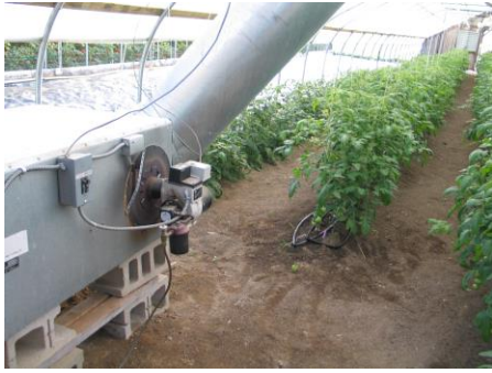
Oil furnace with a Beckett burner in a tomato greenhouse.
