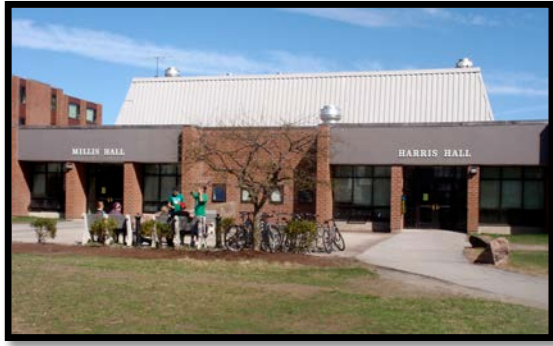
Figure 17. Entrance to Harris-Millis Dining Hall. Photo by Sara Cleaver, 2012.
