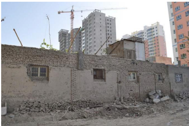
(“The demolition in Hotan”, 2012)
