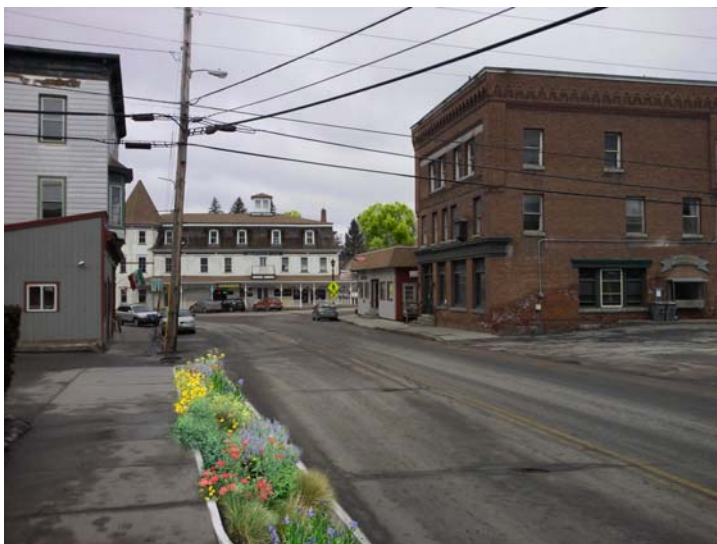
D.1: Perennial species-vegetated bioretention cell with curb cuts to capture and filter stormwater using plants and soil.
