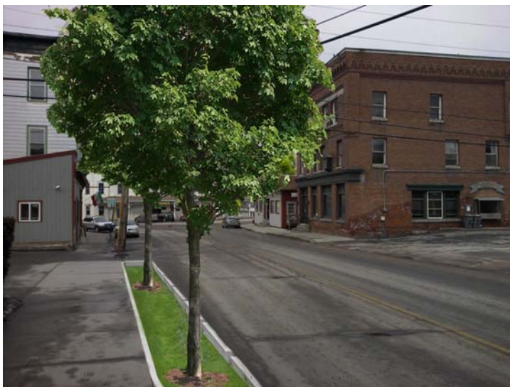
C.1: Grass-and-tree vegetated bioretention cell with curb cuts to capture and filter stormwater using plants and soil.
