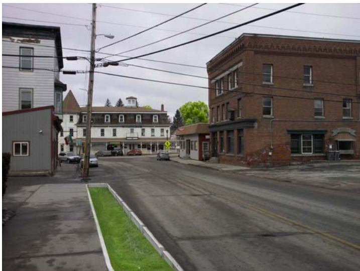
B.1: Grass-vegetated bioretention cell with curb cuts to capture and filter stormwater using plants and soil.
