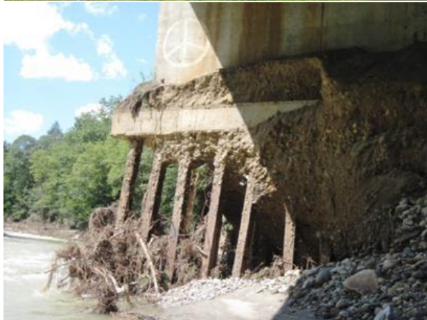
Figure 3.3: Example of flanking (a) and abutment scour (b) damage to bridge embankment and abutment due to Tropical Storm Irene (source: Vermont Agency of Transportation)
